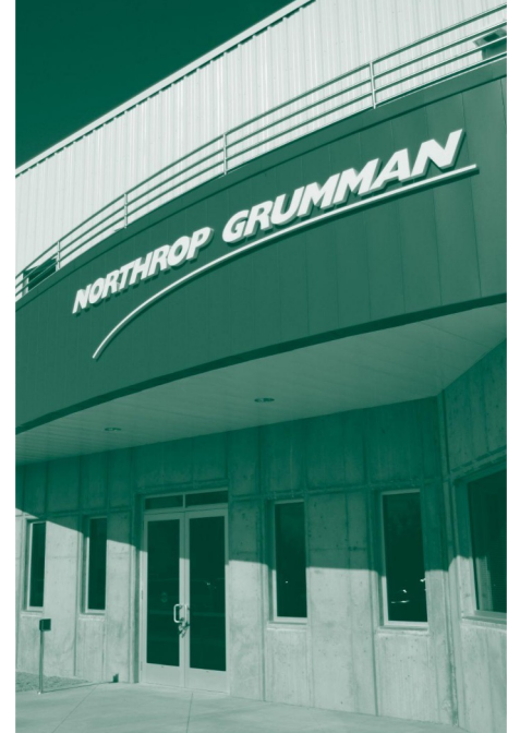
Port Authority Partnership SLC, Northrup Gruman
